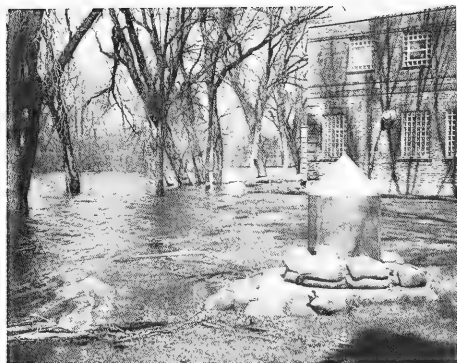
Figure 3.--Water level of 15.4' at the northwest corner of the Laboratory on April 18, .4' under the flood crest of 15.8' which occurred on April 20. Photo taken by Bernard L. Berger.
